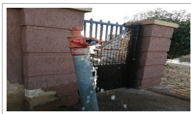
FIGURE 3: Emergency tap leaking in Alabama Street, Extension 16 in Protea Glen.
