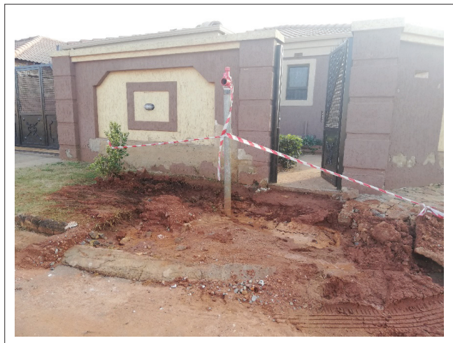
FIGURE 4: Damage caused by the leaking emergency tap in Alabama Street, Extension 16 in Protea Glen.
