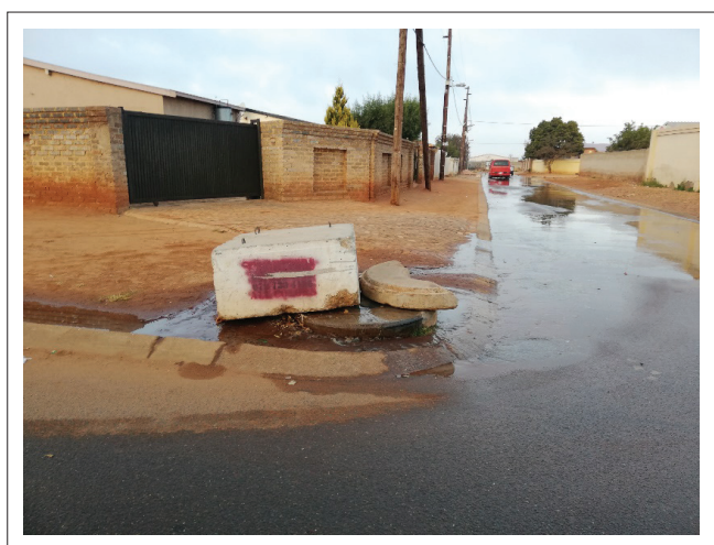
FIGURE 5: Leaking sewerage drain in Alabama Street, Extension 16 in Protea Glen.
